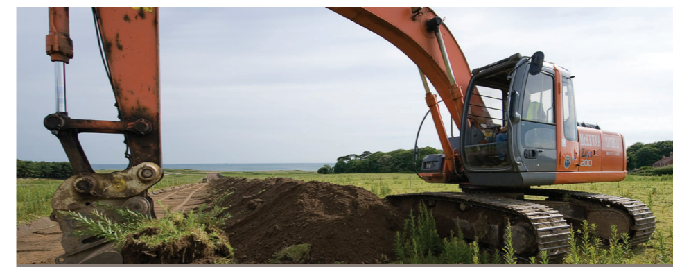
Onshore cable work underway at Weybourne
